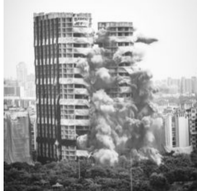
File photo of Supertech's illegal twin towers being razed on August 28
